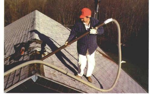
**Filling sloped-ceiling bays with blown cellulose.** The pipe extension on the blower's hose reaches the bottom of the bay, ensuring a dense, air-sealing pack.
