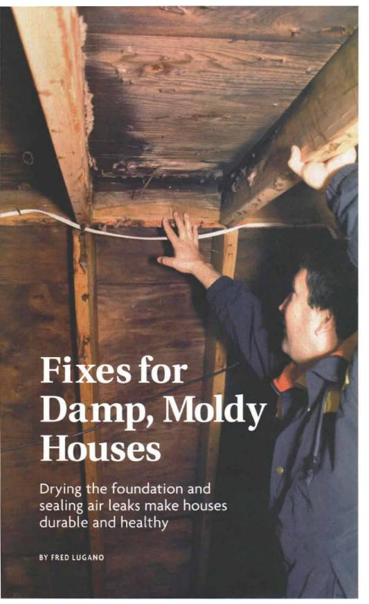
Condensation leads to mold growth and rot in the attic. The moisture source is probably the basement, and leaks in the building shell and in ducts carry the moist air upward.
