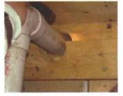
Holes and gaps in the framing pass lots of moisture. Sealing the holes is simple, though. A shot of urethane foam stops the flow of moisture-laden air.
