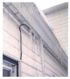
Attic ventilation doesn't always work. Stopping moisture from entering this attic in the first place would have prevented ice from forming.
