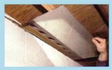
A mirror reveals open block cores, a great moisture source. The fix is easy, though. Cap the cores with expanding foam or simply stuff them with wads of plastic sheet.
