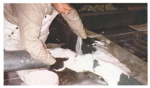
**Duct-sealing is critical.** Unsealed ducts blow hot, moist air into the house's framing cavities, or suck damp air from foundations. By the way, use mastic; duct tape doesn't air-seal.
